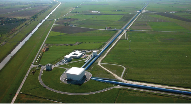
Fig. 1. Aerial view of Virgo detector with the two perpendicular 3-km long arm across the Tuscanian countryside. Credit: The Virgo Collaboration.
