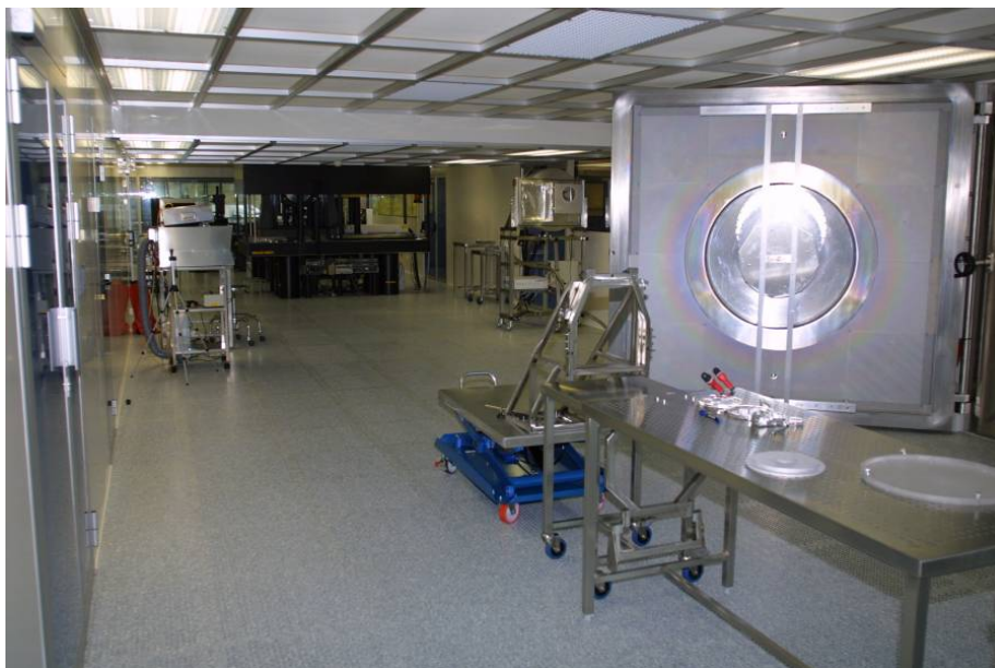
Figure 51. General view of the class 1 clean room (surface: 150 m 2 ).
